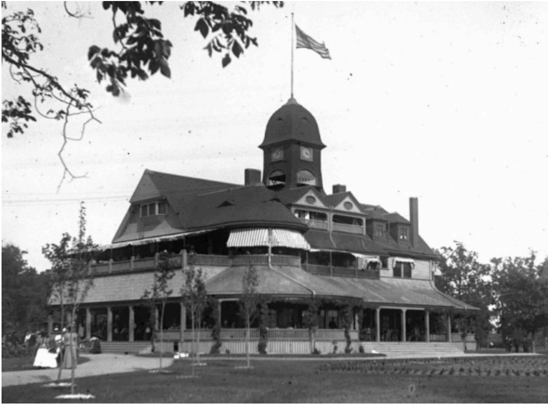
Figure 5.6: The old casino on Belle Isle demolished in 1908 (Burton Historical Collection, Detroit Public Library)
