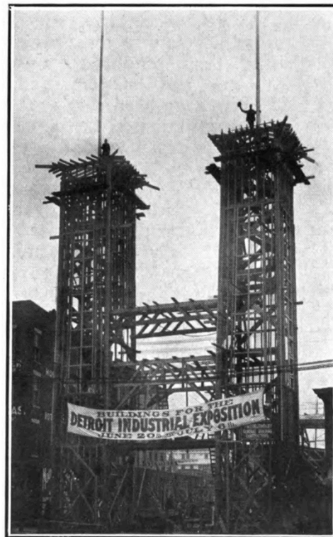
Figure 5.11: The Exposition Building under construction with two workers standing on top (Souvenir of the Detroit Industrial Exposition)
