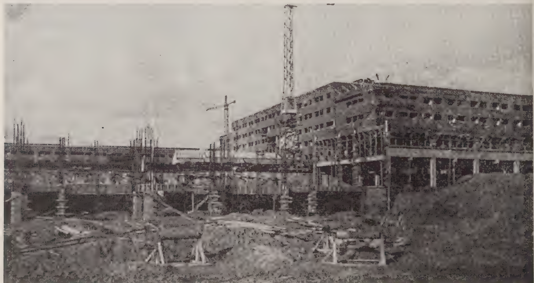
▲ Madrid: City University — Clinical Hospital construction site. Scene of bitter fighting
